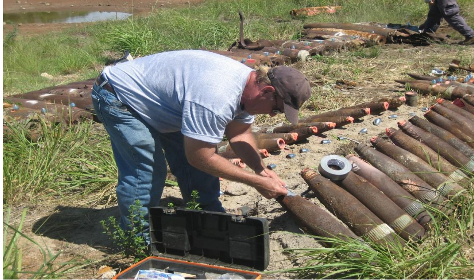
Figure 3.3. Consolidation of UXO items and preparation of explosive demolition
